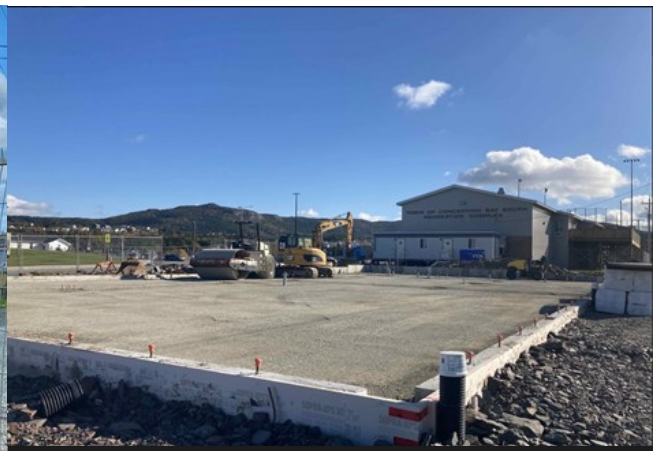
The construction site of the new CBS Public Library
