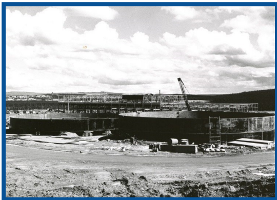
Wabush mines - 2 10,000,000 gallon water tanks & crusher. Perlin Collection PA1514, C422.
